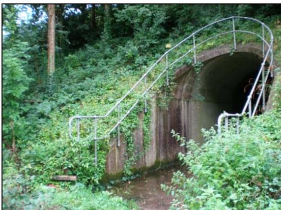
Undergrowth surrounding the tunnels causes water to run onto the concrete floor.
