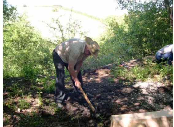
Excavating holes for the bench legs.
